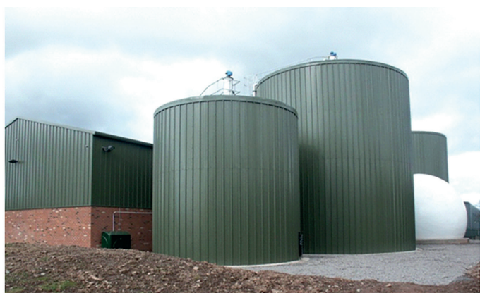
900 m 3 mesophilic digester, buffer tank, gas storage and digestate storage at the South Shropshire plant
