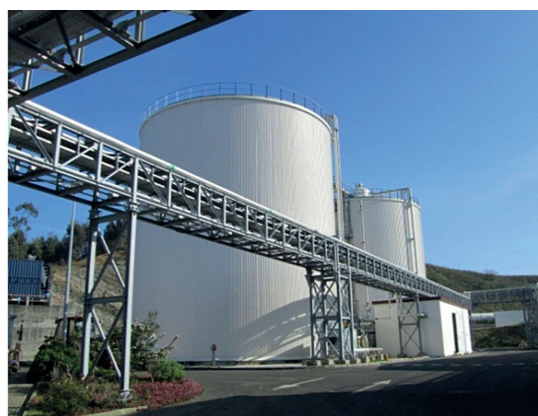
Two 3500 m 3 thermophilic digesters at the Valorsul AD plant in Lisbon
